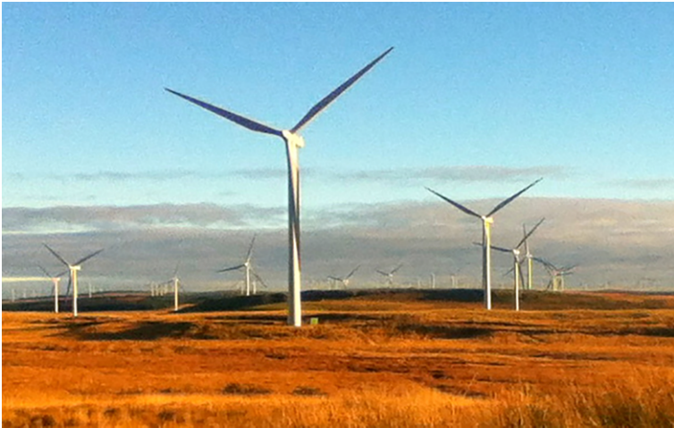
Figure 8.11 Whitelee Wind Farm, Scotland (Source: personal photo, author).
