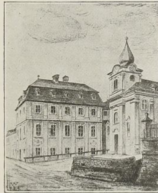
Körnerhaus in Döbling.
