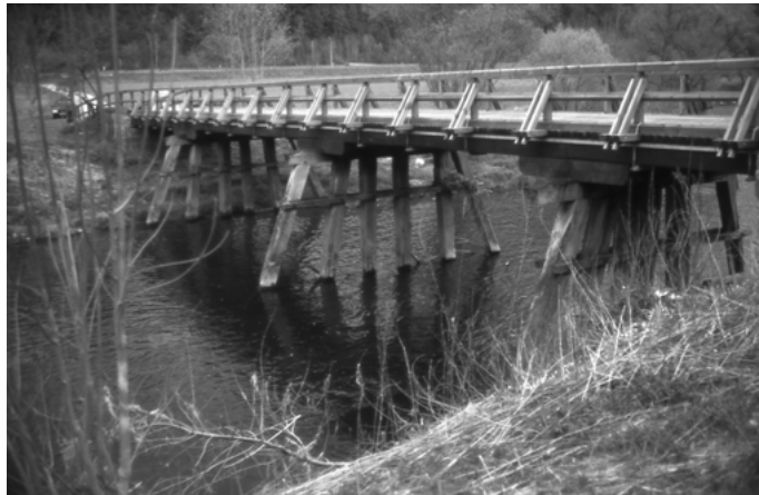
Fig. 7: Neckarhausen, bridge built 1257.
